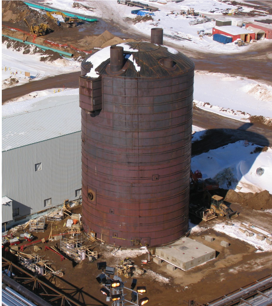
Figure 1: Hot water tank
