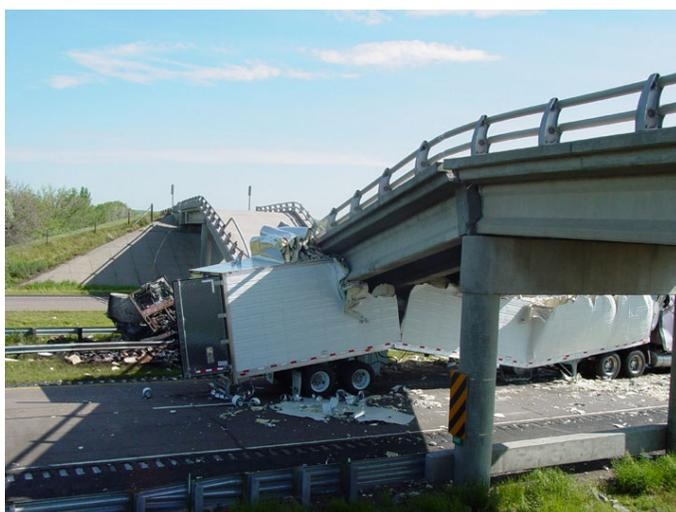
**Figure 2:** Collapse of I-80, Nebraska, bridge after being struck by tractor trailer (courtesy of NDOR)
