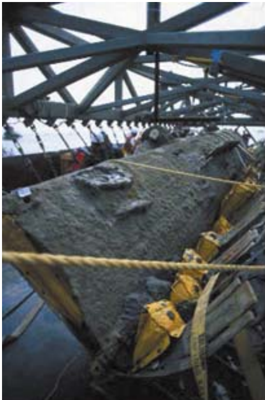
In the recovery of the Hunley, 32 slings attached to a steel frame supported the vessel's 65,000 pounds as a crane lifted the submarine to the surface.
