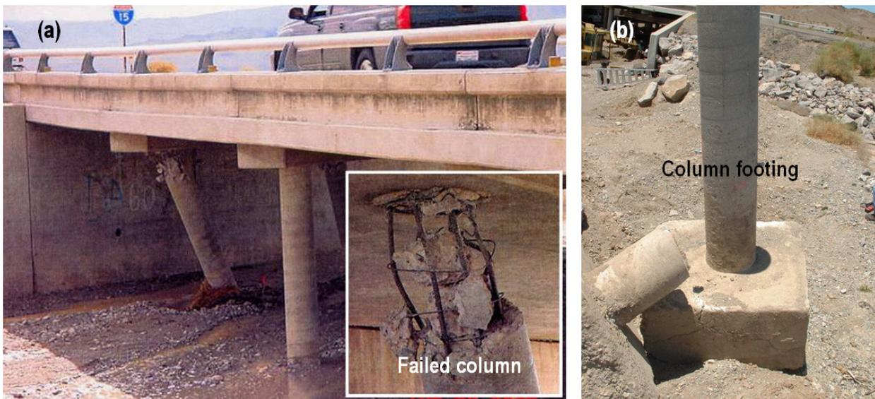
Figure 1: Oat Ditch Bridge on I-15 in California (a) failed column (b) column footing
