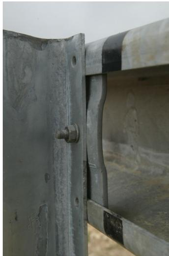
**FIGURE 5** Post to rail attachment using clamp plate connection.
