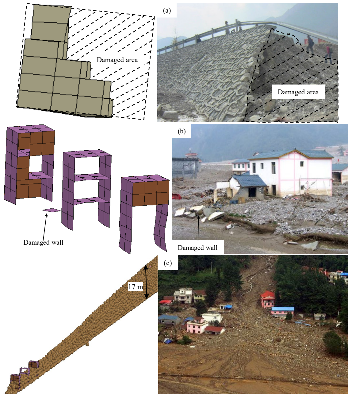
Fig. 7 Comparative analysis with the actual situation (a) damaged dam, (b) damaged houses, and (c) deposition height
