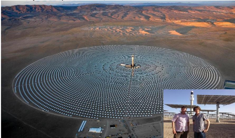
Fig. 1: The Crescent Dunes tower CSP plant with 1.2 million m<sup>2</sup> aperture area [1, 2].
