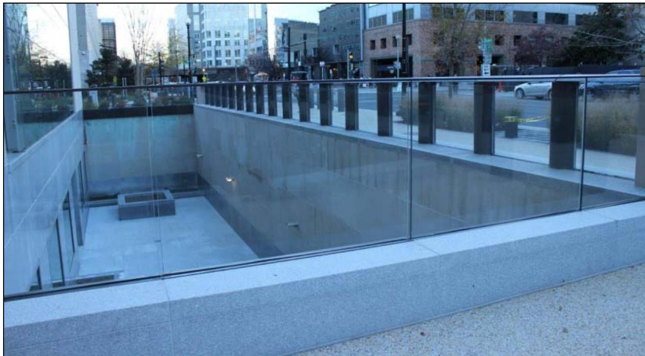
**Figure 11 – Final Construction of VBIED Perimeter Protection Installed at Top of Subgrade Courtyard**
