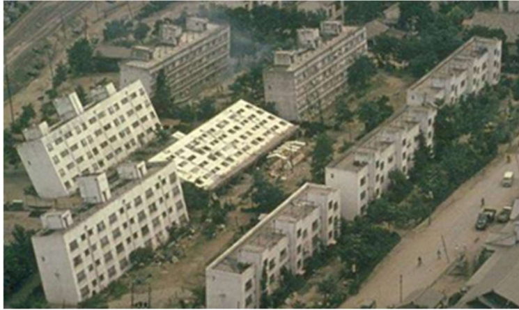
Fig.1: Collapse of apartment blocks caused by liquefaction in the 1964 Niigata earthquake
