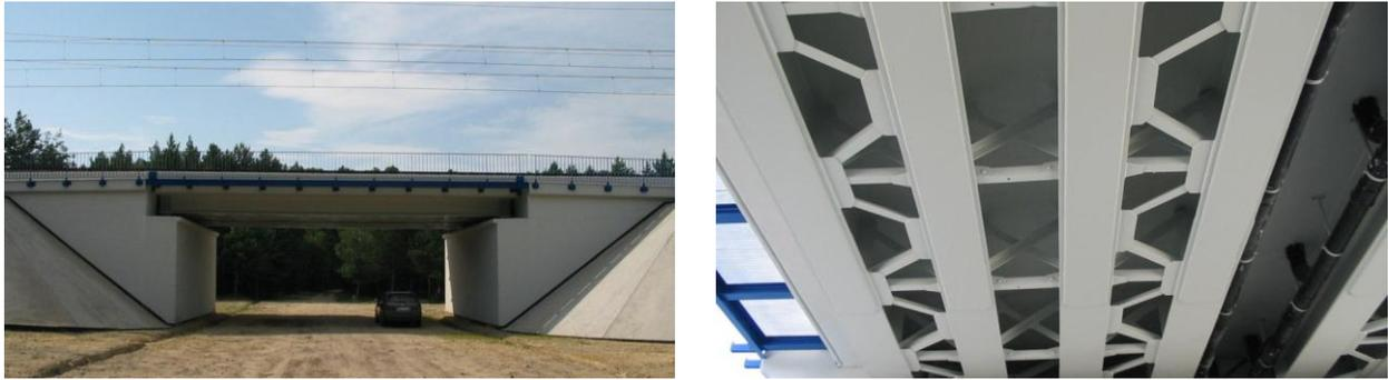
**Figure 1:** The modernized viaduct No. KNI 140070 composed of two separate spans, located at 200.794 km on the PCML — a side view (*left*) and view on the main steel beams with the bracing system (*right*)
