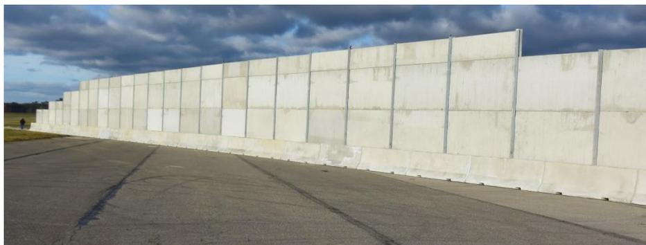
Fig.1: Portable road barrier with integrated anti-noise wall
