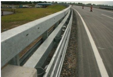
Fig. 1: Vehicle restraint system.
