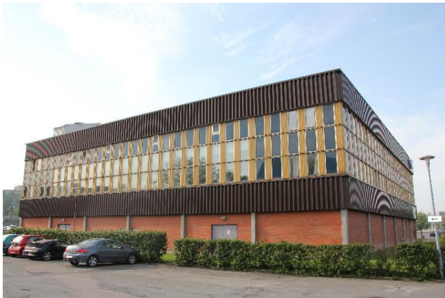
Fig.3: Gompute Data Center, Gothenburg (Sweden)
