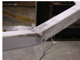
b) Buckling of brace
