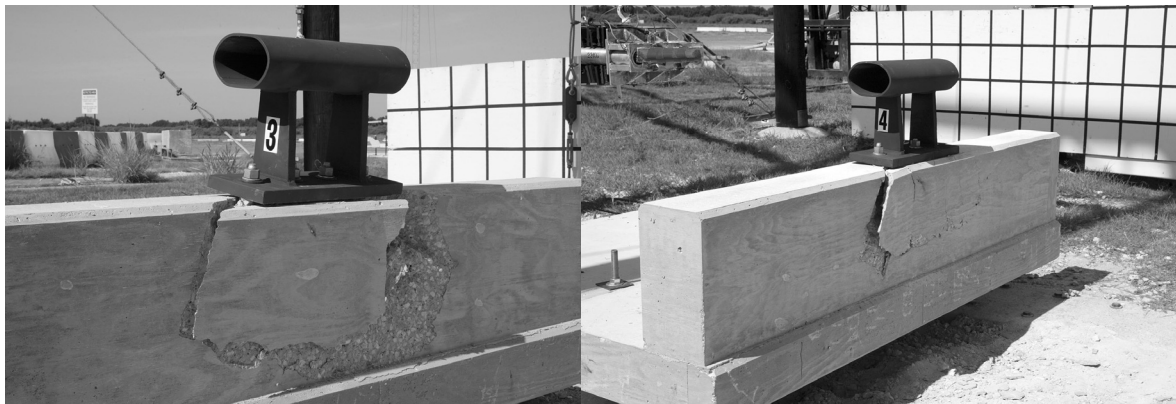
Figure 3 Parapet damage after test P3 and P4.
