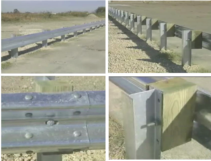
Figure 1: Typical W-Beam Guard Rail System
