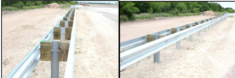
Figure 16 TxDOT 31-inch W-beam median barrier installation
