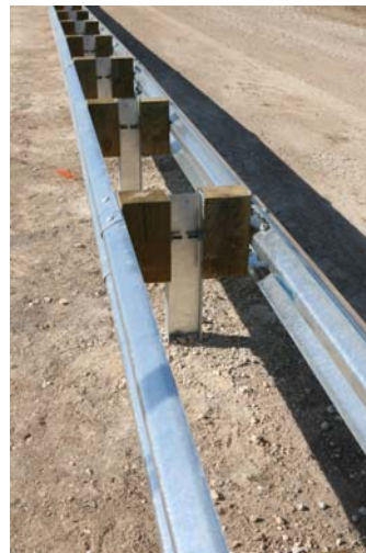
Figure 6 Cross-section of a 27 in W-beam median barrier
